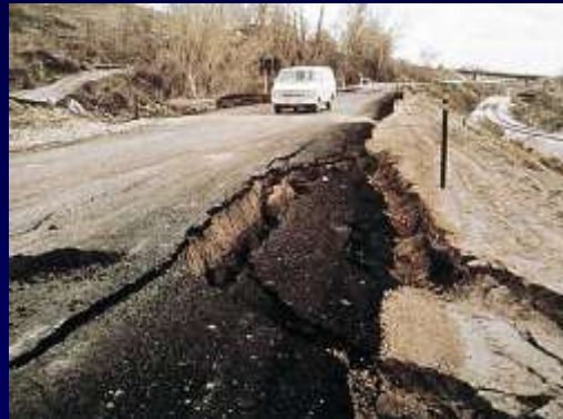
Road destroyed by swelling clays
